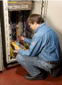
**Troubleshooting tools** - electrical scopes, digital multi-meters, insulation testers
