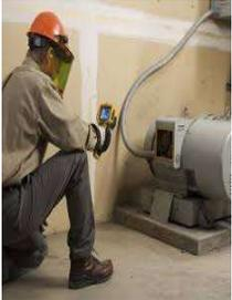
**Screening tools** - thermal imagers, vibration meters, vibration sensors
