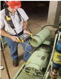
**Predictive tools** - vibration tester, vibration analyzer, corrective tools, vibration sensors
